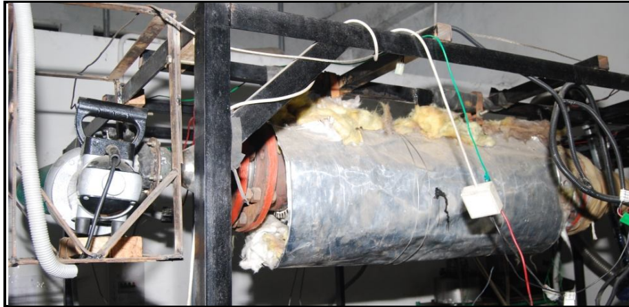
Figure 3.35: Electrically air preheating system.
